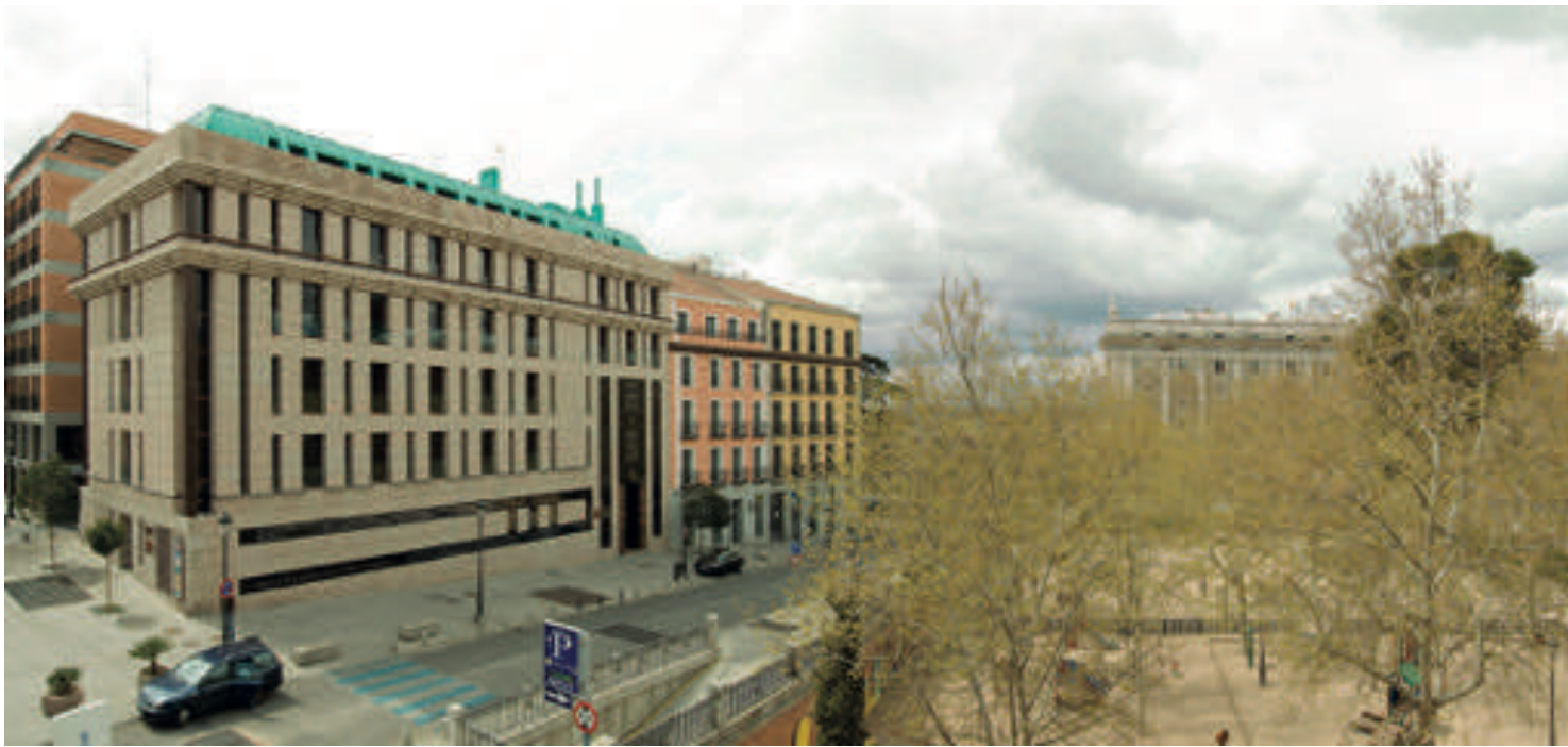
The Reina Sofia School of Music: building by architect Miguel de Oriol, at the Plaza de Oriente in Madrid.
